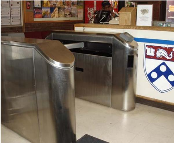
These high-security turnstiles utilize card readers and keypads to allow for a dual-technology entry system. The first step is to swipe the access card. Then a unique, four-digit code is entered. The card reader/keypad is tied into the university’s access control system. In addition, two CCTV cameras with opposing views are aimed at each lane, and all camera video is recorded 24/7. In the event of an alarm, the associated camera frame rate increases.
